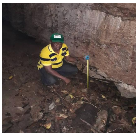
Figure 16: Cliff foot formed at the base of a cave wall
