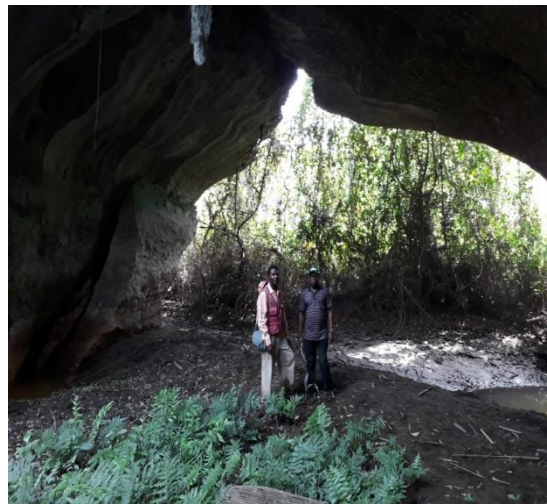
Figure 15: Corrosion bridge at the base of a bluff at as Abung
